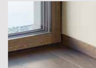
Skirting board with flush wall termination
